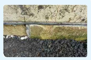
A damp-proof course (DPC) is a barrier in a masonry wall designed to resist moisture rising through the structure. Be careful not to allow the damp proof course to become bridged by the build up of plants and soil, or by building a patio.
